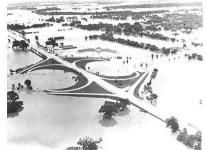
Flooding in northeast Topeka, 1951
